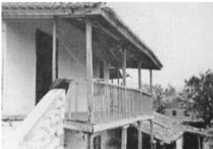
A house on the hills of Ghana in Africa... or a house in Siatista, northern Greece... and a house in Fychtia in the plain of Argolis in Greece, look as if they were the work of the same builder
